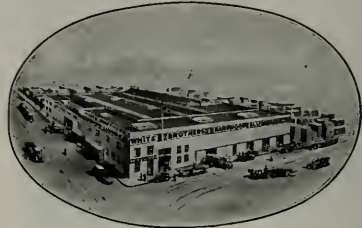
Present plant at 5th and Brannan Streets, San Francisco.
